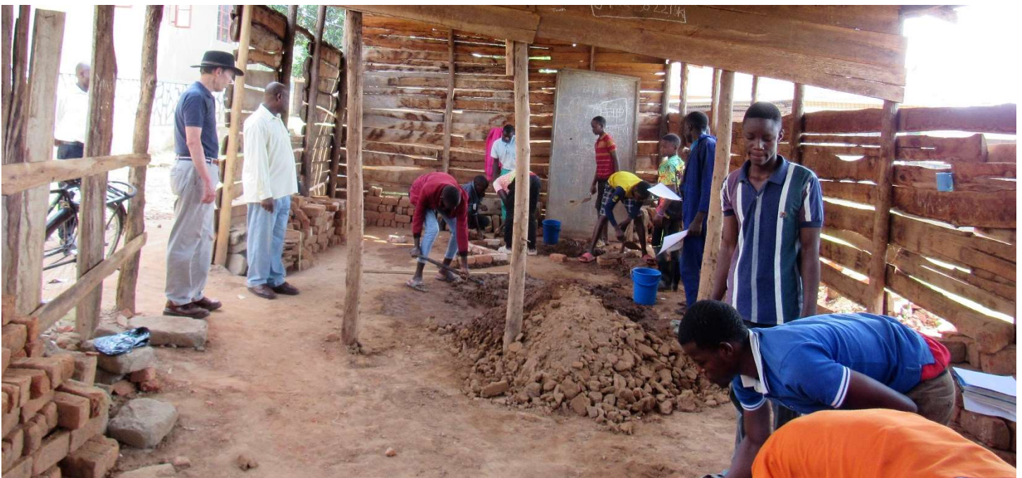
Young men learning how to make bricks in the construction class
